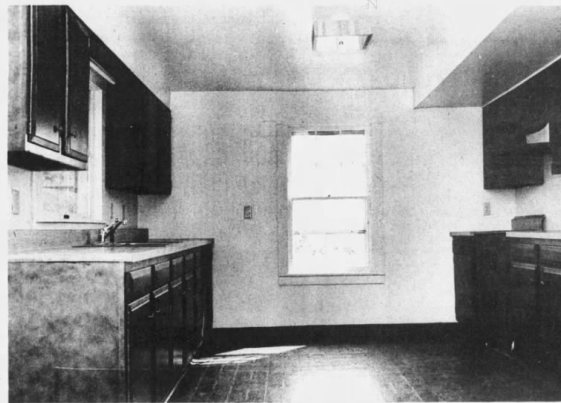
The large kitchen has been completely remodeled with the installation of modern cabinets, new lighting fixtures and new floor covering.
