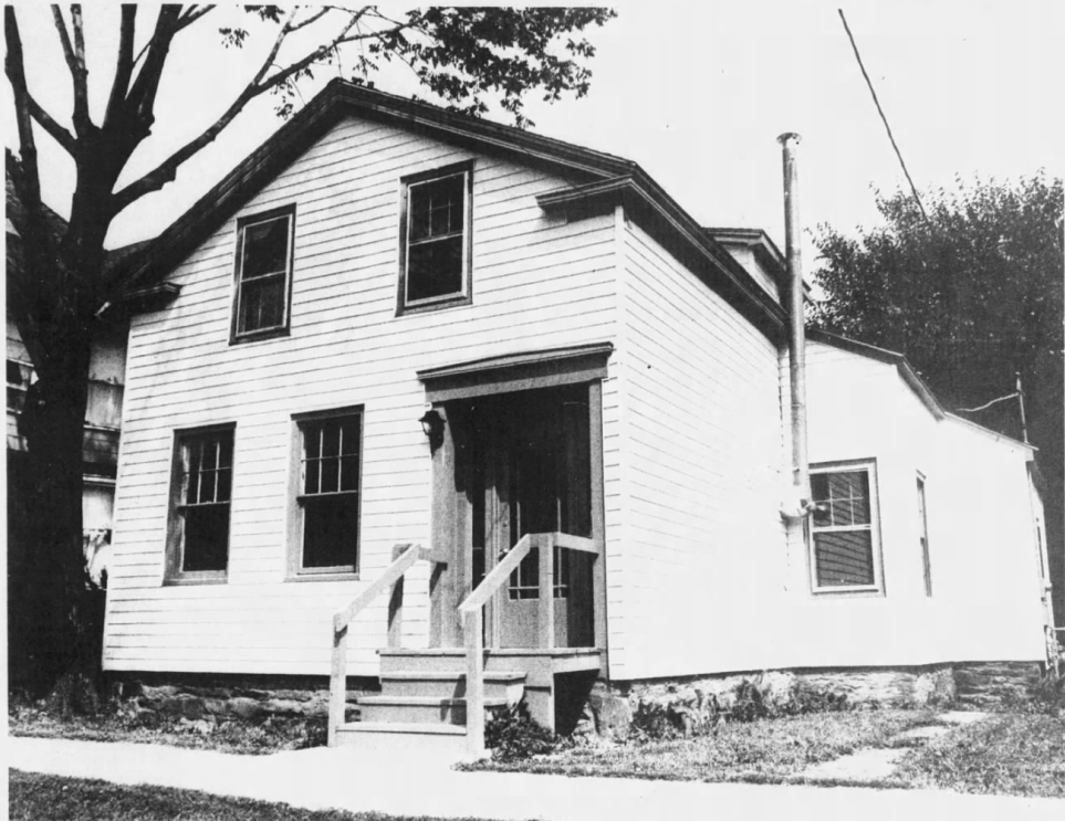
The City of Ithaca has remodeled this house at 213 S. Plain St.
