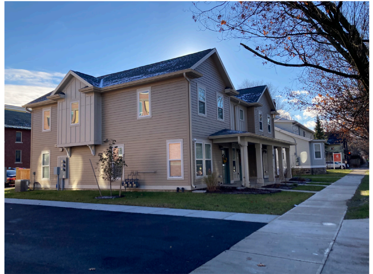
307 N Plain townhome, new construction (#6 on aerial).
