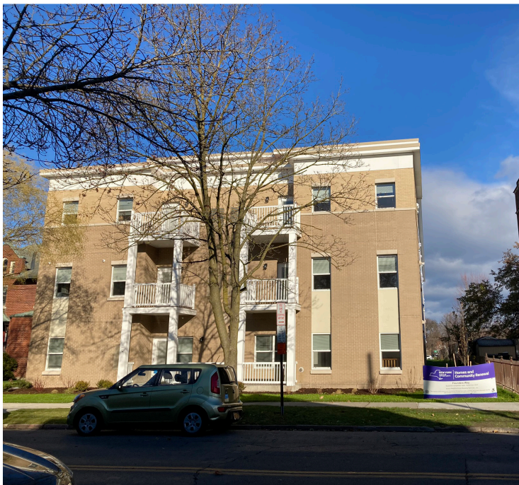
AFTER: South Wing from W. Buffalo St.
