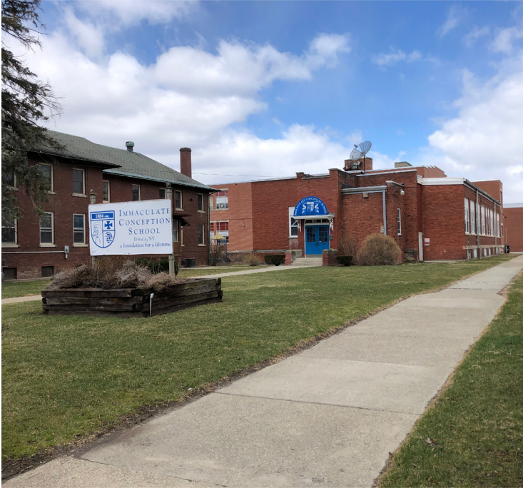
BEFORE: South Wing from W. Buffalo St.
